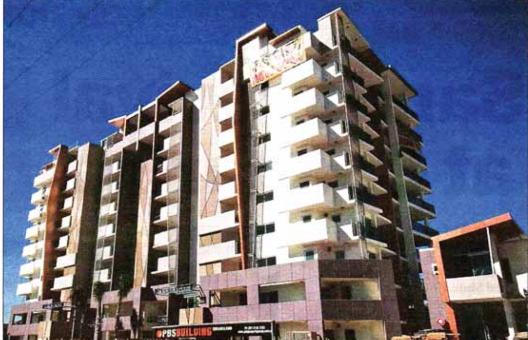
Modena on Chevron is two-thirds sold ahead of its completion next month (above) and a concept image of the project (below)
